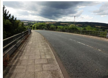
3. View of carriageway looking West
