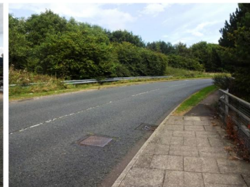
4. View of carriageway looking NE
