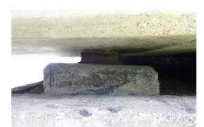
17. Typical view of bearing
